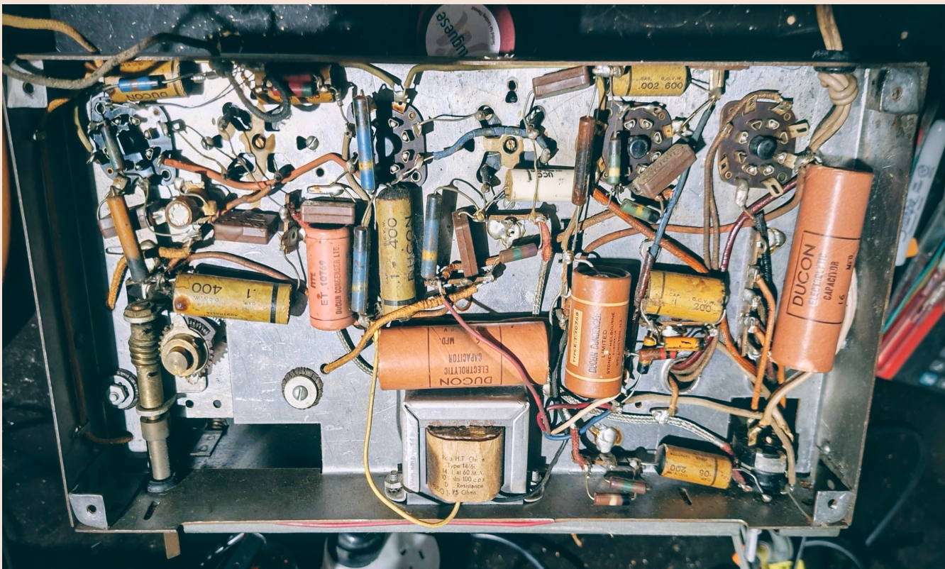
Fig 5. After full service and replacement parts into original housing and layout.
